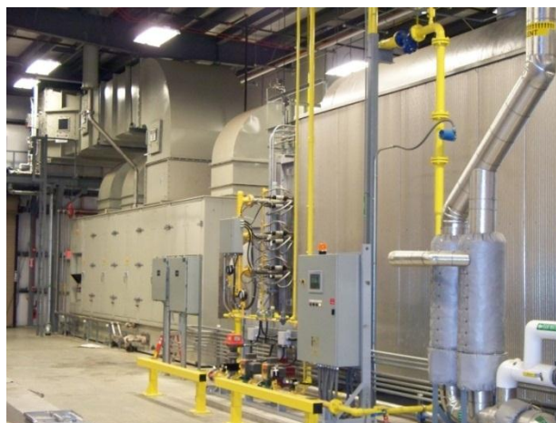
Figure 1. A typical 1.5 MW gas turbine CHP system
