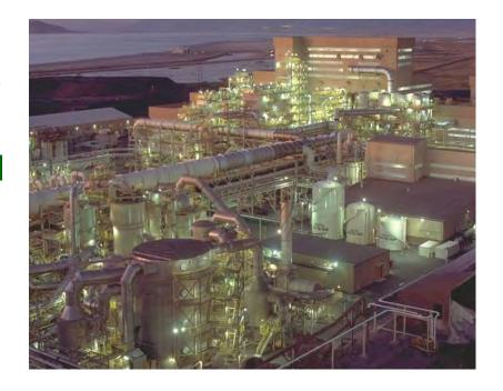
natural gas burners) and added to supplemental steam from two other gas-fired boilers as necessary to drive the acid plant compressors. The compressors pull the emissions through the pollution control equipment upstream of the compressors and then push the gases through the downstream acid plant. Heat is captured from the exothermic (heat producing) conversion of sulfur dioxide to sulfuric acid to produce yet more steam.
